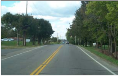
View looking north on SR 48
